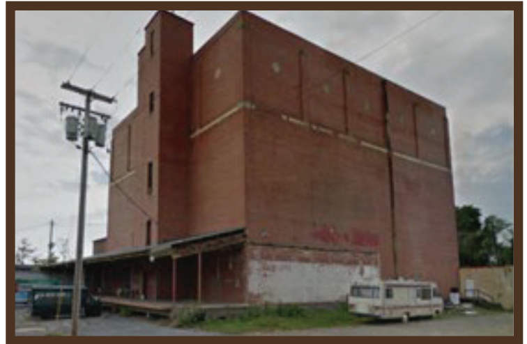
Former Building Demolished.
